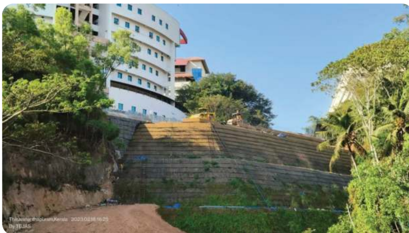
Figure 4. Coir Geotextile as one of the components of vegetated facia units for construction of 27m high reinforced soil structure at Technopark, Trivandrum, Kerala
